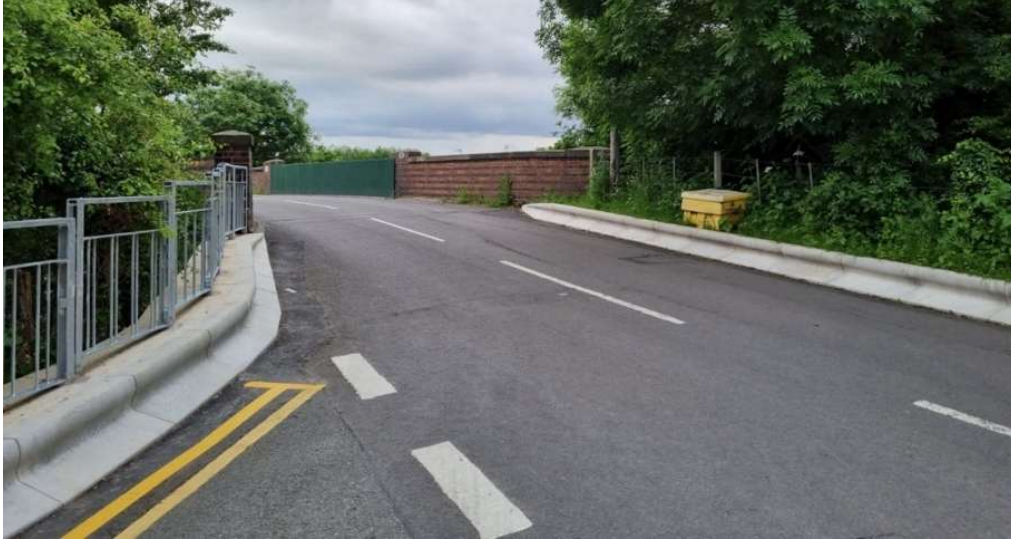
Rail bridge Hatton Station looking south from Station Approach
