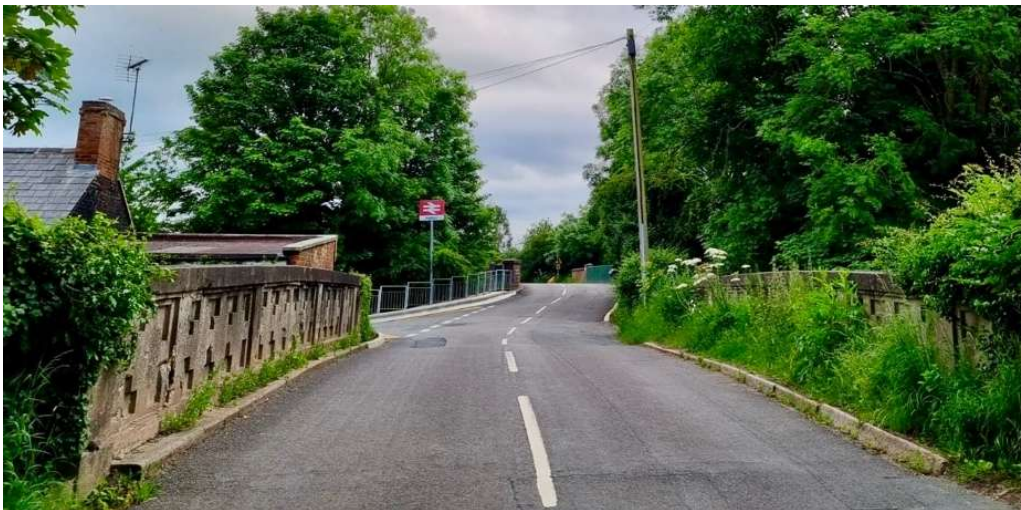
Station Road (D50930) looking south across canal bridge to station access road on left and road over bridge beyond.
