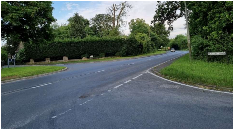
A4177 / B4439 Hockley Road junction looking towards Warwick
