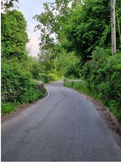
Dark Lane looking northwards towards canal bridge
