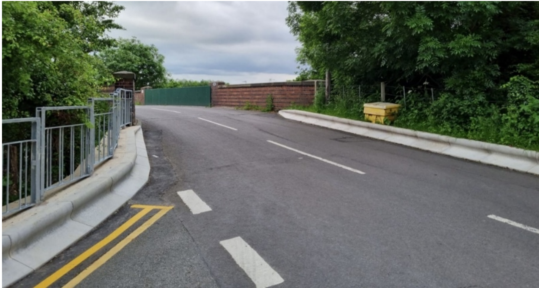
Rail bridge Hatton Station looking south from Station Approach
