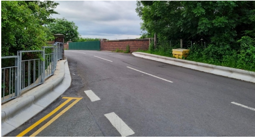
View from Station Approach looking South
