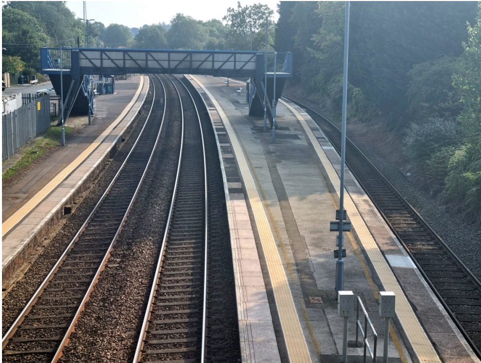
Hatton Station, looking towards Leamington, showing Platforms 1,2 & 3
