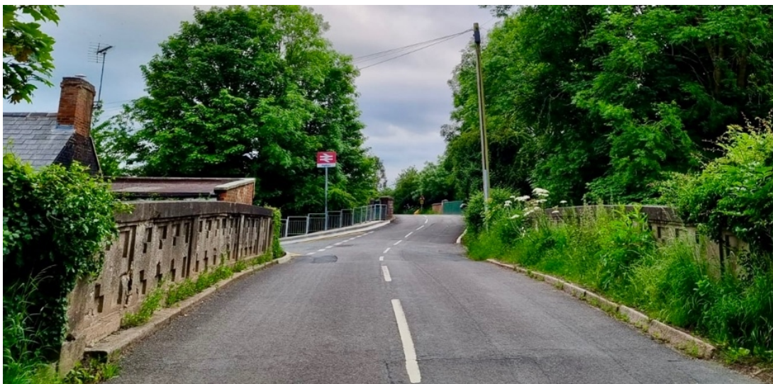
Station Road (D50930) looking south across canal bridge to station access road on left and road over bridge beyond.
